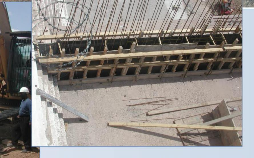
The spillway was painted with PVA to reduce the rate of drying of the concrete.
