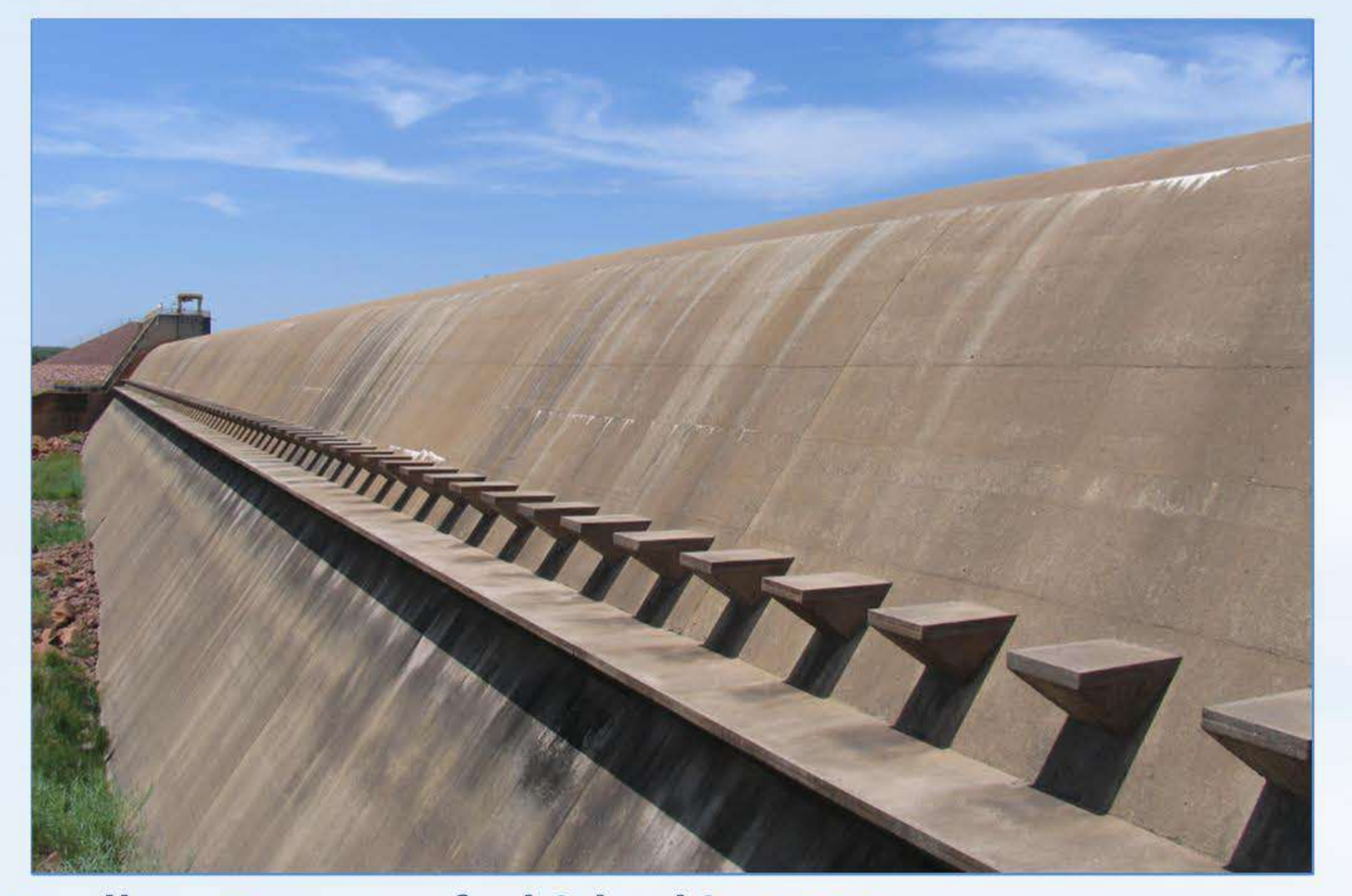
Vaalkop Dam – refurbished in 2008 (Photo: DWS)
